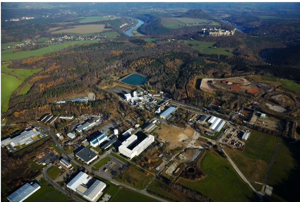
Figure 3-19. Aerial view of the Königstein operation plant.
