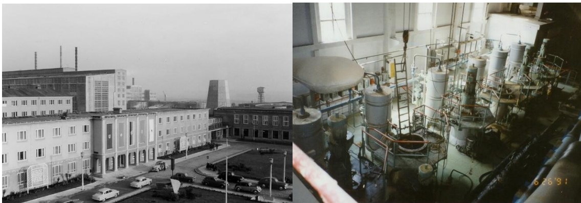
Figure 3-21. Seelingstädt operative plant
