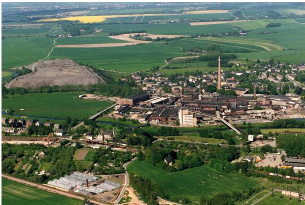
Figure 3-22. Facilities of the operative plant Crossen with the dump of mining residues
