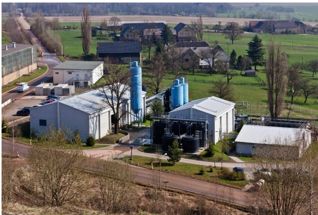
Figure 4-22. Water treatment plant WTP in Seelingstädt
