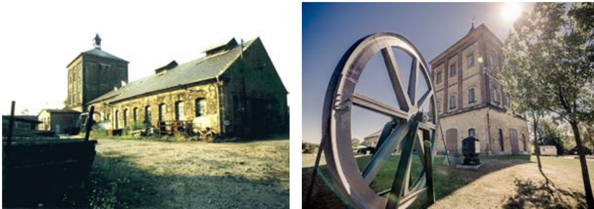
Figure 4-13. Shaft building of the Marienschacht with Malakoff winding tower, 1886 and in the 1990th
