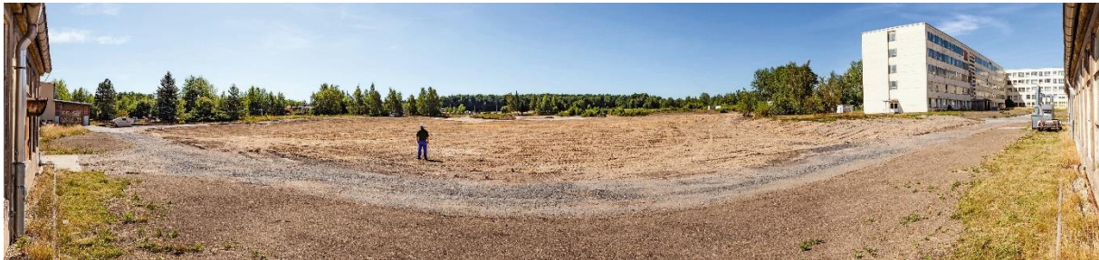
Figure 4-40. Rehabilitated area of the shaft complex 388/390 at Königstein site in 2015.
