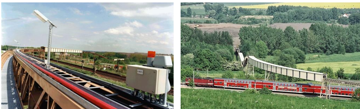
Figure 4-17. Transport of Crossen mining waste and processing residues to the industrial settling plant Helmsdorf with Pipe Conveyor
