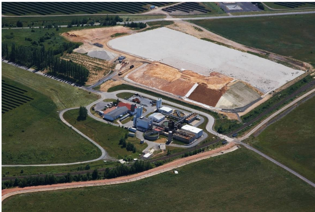
Figure 4-24. Water treatment plant WTP in Ronneburg with the area for storage of immobilized pollutants behind.
