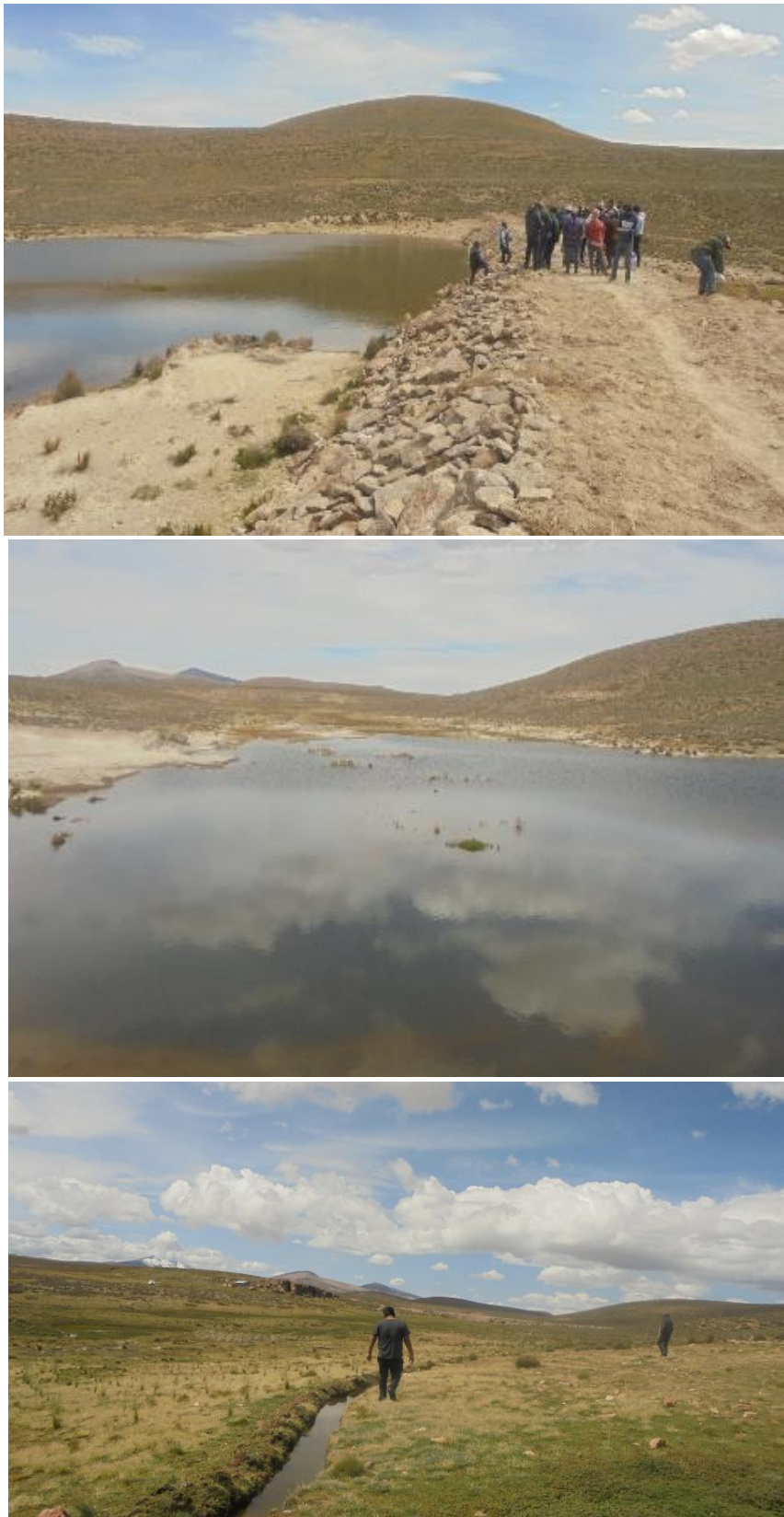
Figure 5-10. Micro-dam project within the properties of Mrs. Brigida Up: Microdam wall. Middle: Collected water. Down: Channel and improved lands.
