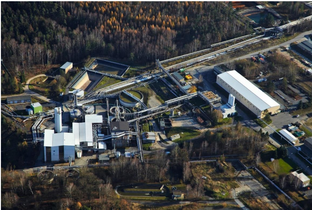
Figure 4-12. Treatment plant for flooding water Königstein in the state of 2015, which was modernized in 2020.
