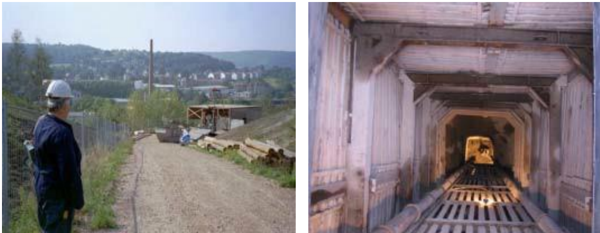
Figure 4-14. safekeeping of the “Schurfschacht 60” in 2002
